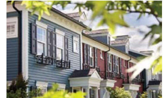
Articulated elevations add richness to building exteriors.
